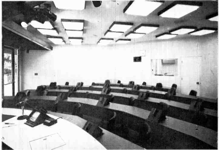
Fig. 5. A view from the front of the TV studio classroom. At the front can be seen the lecturer's monitor and microphone; similar units are positioned between each two students. The control room window is at the rear, to the left of which is the rear-mounted camera.
