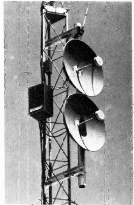
Fig. 6. A receiving location aerial tower. The lower dish is used for TV pick-up and is connected to the down-converter bolted to the tower. The upper dish is used for the audio talk-back transmission.
